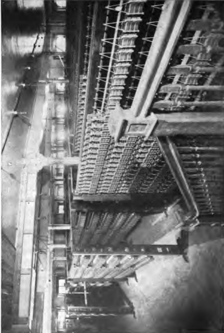
SWITCHBOARD OF AUTOMATIC EXCHANGE OF TELEPHONE DEPARTMENT, CHICAGO SUBWAY CO. Automatic Electric Co.
