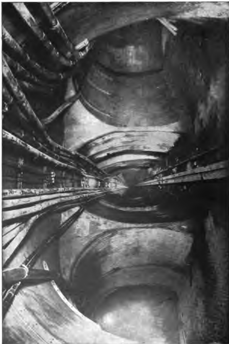
VIEW OF THE TUNNELS OF THE CHICAGO SUBWAY COMPANY. Showing Manner of Hanging Automatic Telephone Cables.
