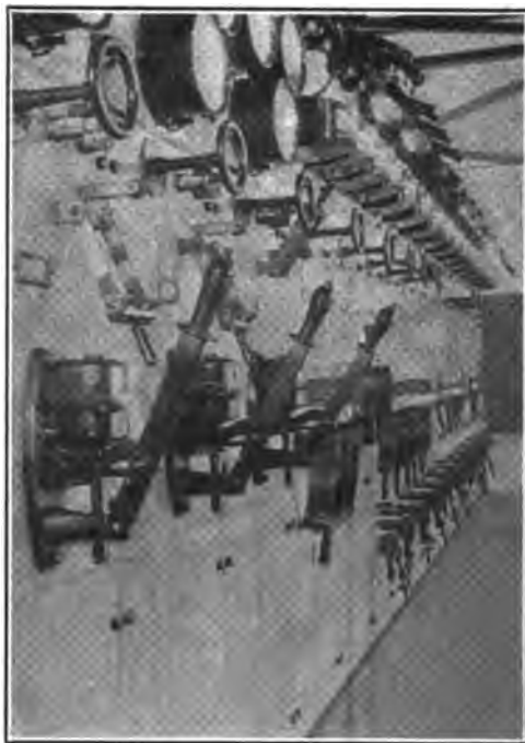
Fig. 308—The Switchboard of the New Brunswick High Power Transoceanic Station.
