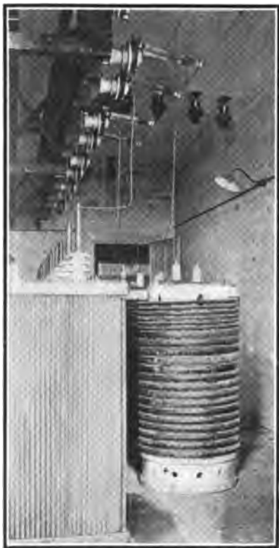
Fig. 307—Bank of High Voltage Trans- formers at Carnarvon Station.
