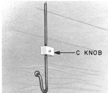
Fig. 2 — C Knob Used As Last Attachment
